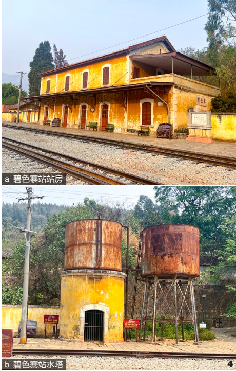
图4 一级站点聚落建筑及附属设施留存情况 Fig. 4 Preservation of primary station settlements and associated facilities
